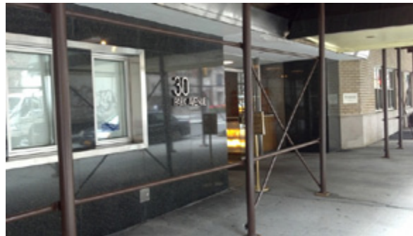
Despite complaints about 30 Park Avenue, no violations were discovered.
